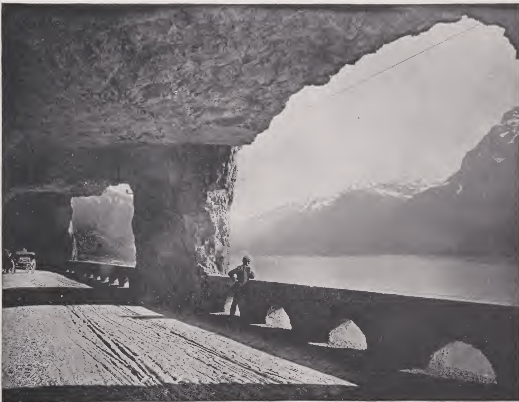
AXENSTRASSE, SWITZERLAND.—This famous road extends nine miles along the Lake of Uri, from Brunnen to Fluelen, and is noted for the remarkable boldness displayed in its construction. It is to a great extent hewn out of solid rock, cut like a shelf into the side of the mountain, with occasional pillars to hold the thousands of tons of rock above, and a strong balustrade to guard travellers from tumbling over the abrupt precipice into the lake many feet below. It is the great highway leading from Switzerland to Italy, and is regarded as one of the most picturesque roads in the world.
